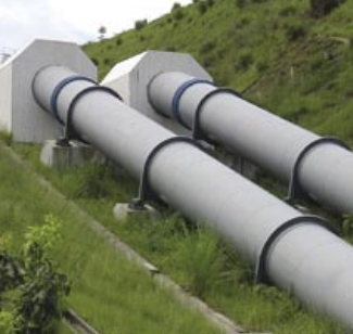
Water Infrastructure Projects in China
